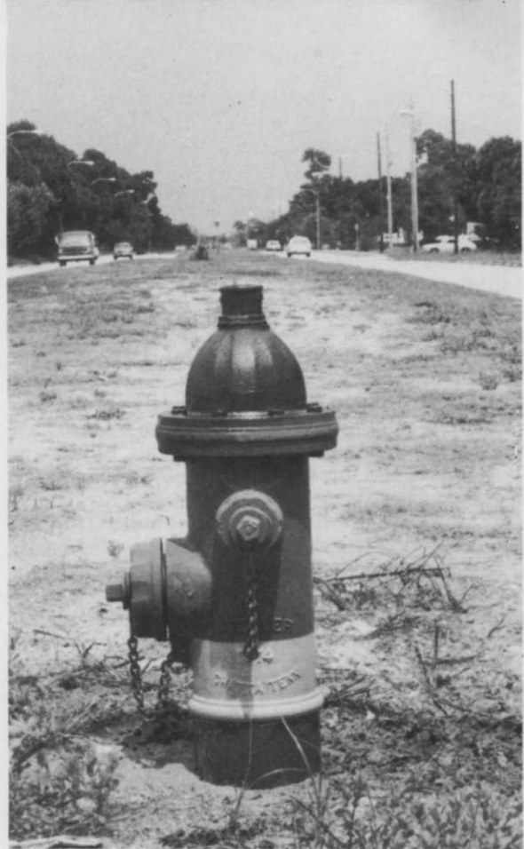
One of the many outlets to the 14-mile distribution system for the recycled wastewater.
