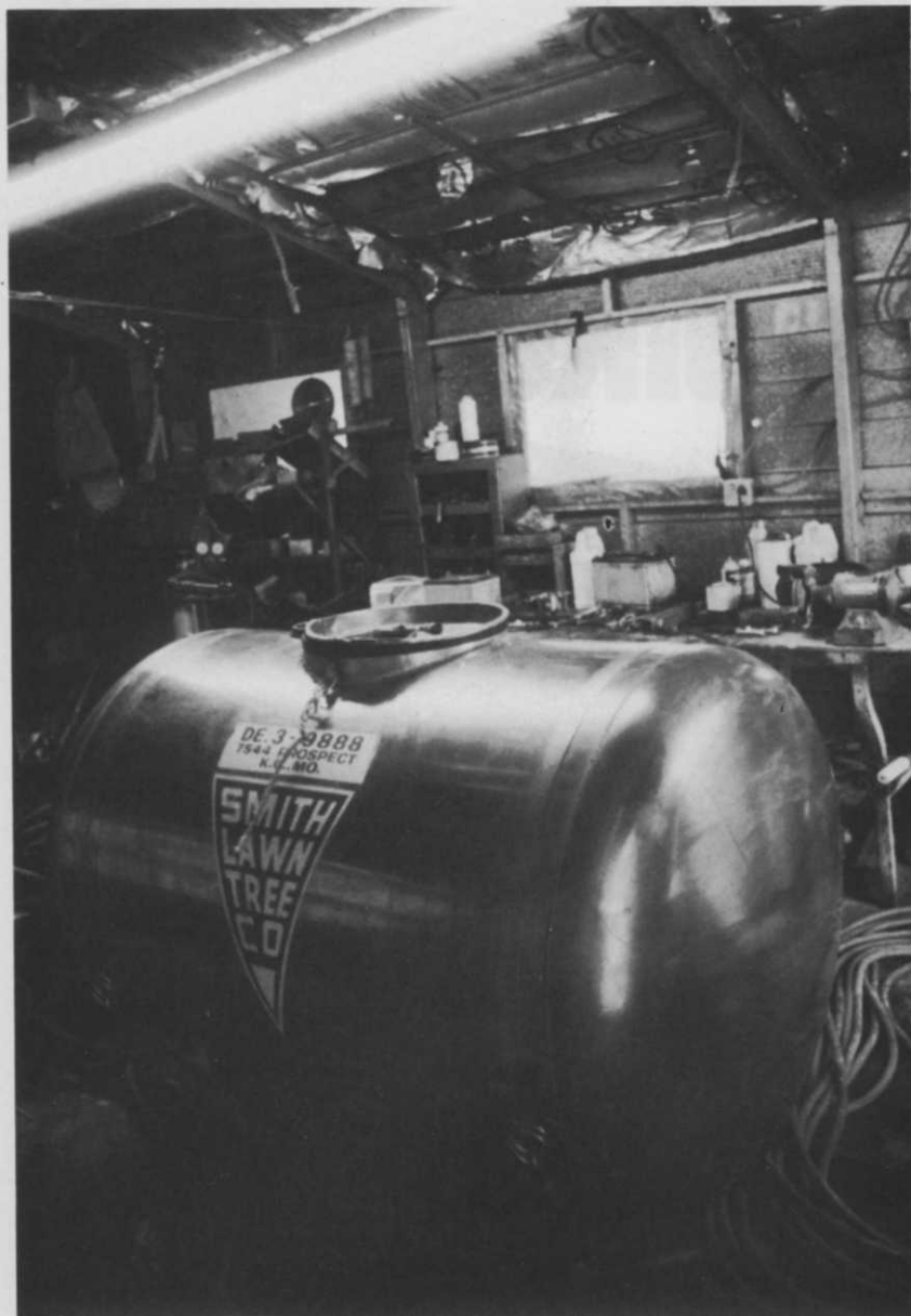
This 300-gallon spray tank, custom made for the firm by a Kansas City manufacturer, is rigged with motor and pump for 400 pounds of pressure.
