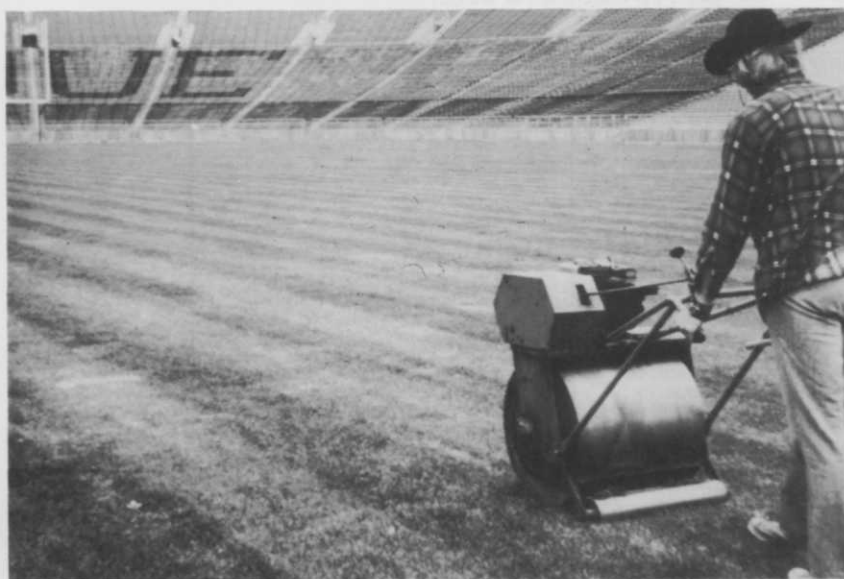
After the sod is put down, it is lightly rolled. The PAT system does not have a crown.
