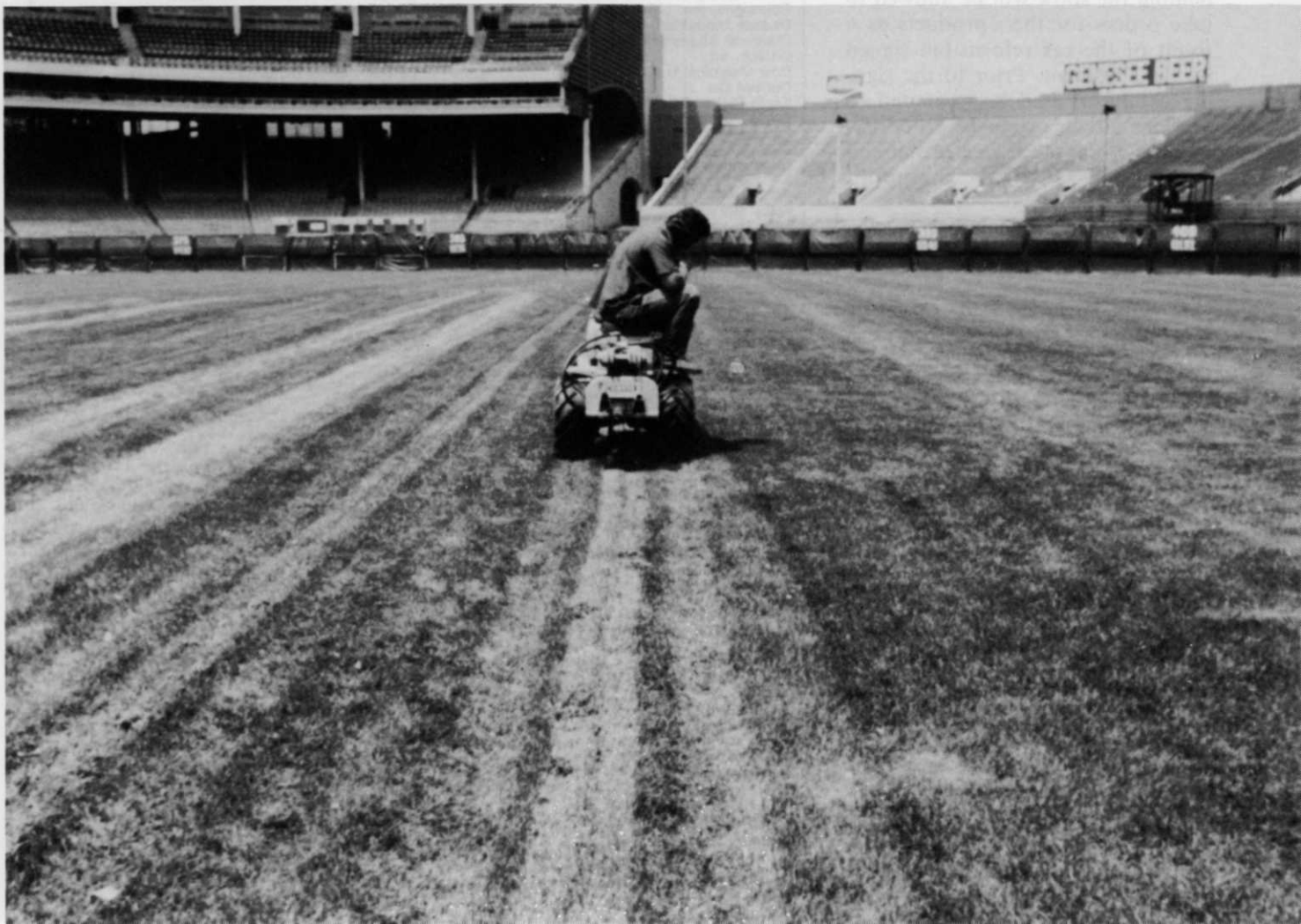
Installation in progress at Cleveland Stadium.
