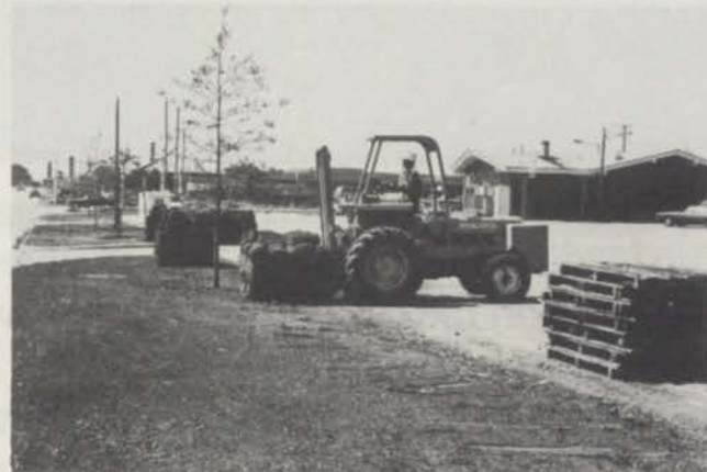
Forklift picks up a fresh pallet of sod to carry 200 yards up the road to installers.
