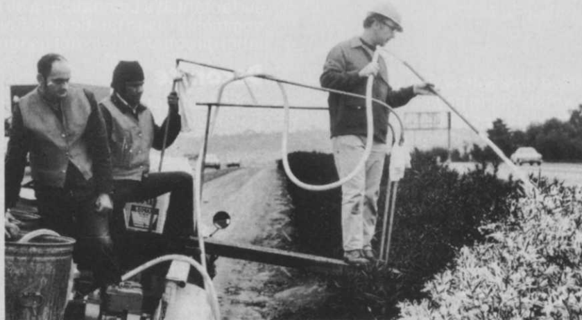
Foam application of Alar on a freeway median planting of Oleander. The foam expansion is by a Waukeshau foam generator.
