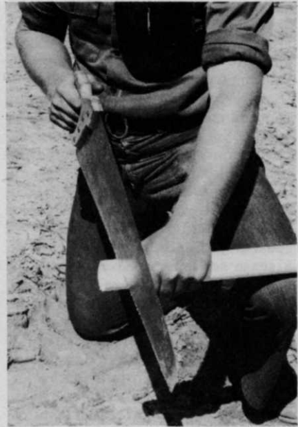
Using PVC for the pipe network also meant the irrigation contractor was able to make length adjustments easily.
