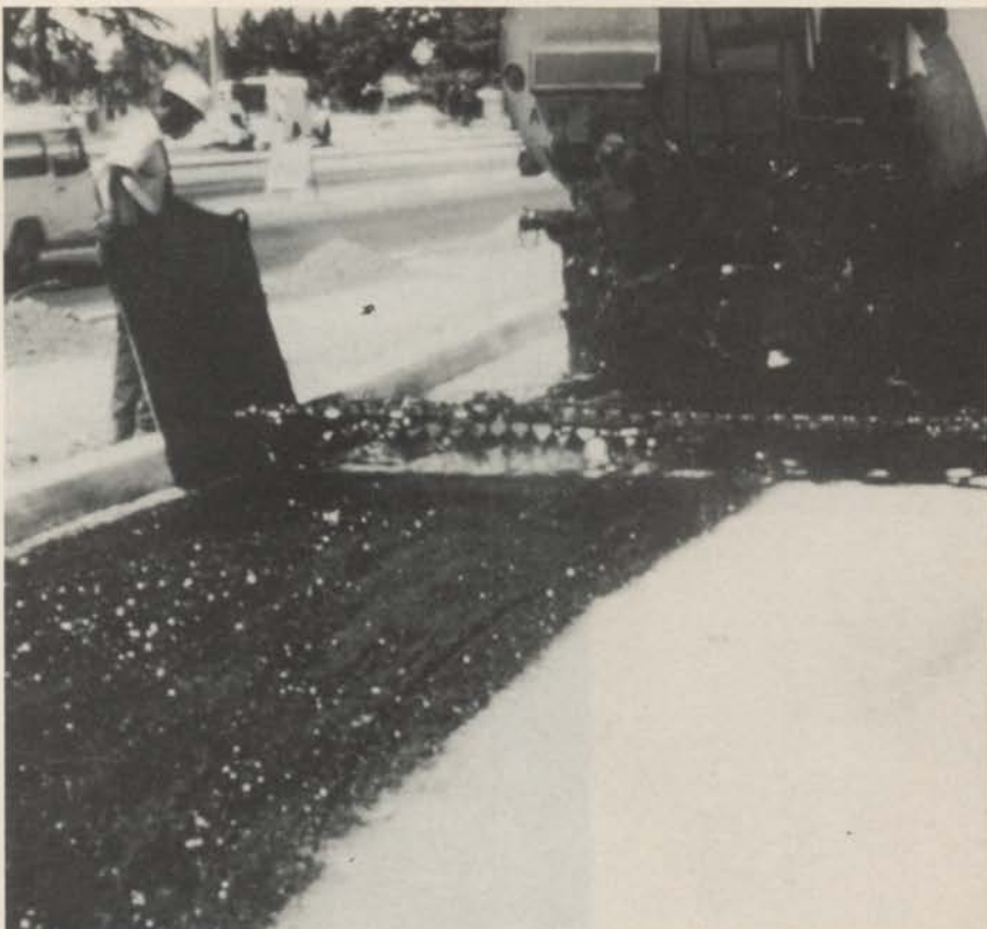
Just ten hours after application of the herbicide, the paving contractor for the parking lot spread a 1/8 inch oil base to seal the soil and trap the herbicide vapor barrier.
