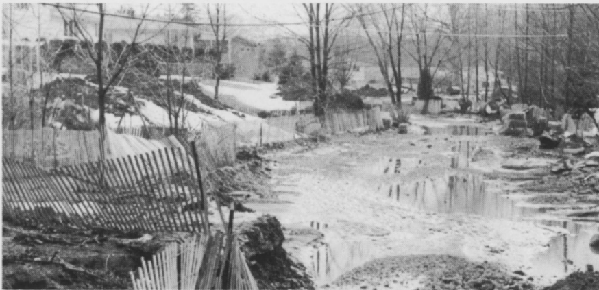
The same area during construction.
