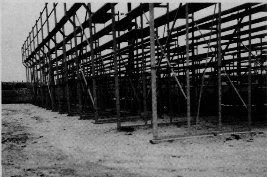
Clean ground under ball park bleachers is treated with Hyvar X. Area is easier to keep clean and tidy when weeds and grass are eliminated. A single treatment lasts a season.
