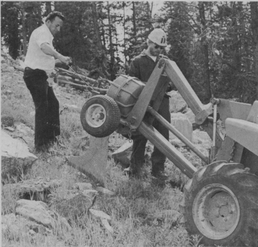
Cable is fed into plow blade.
