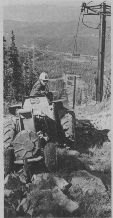
Operator breaks up rocks in first pass.
