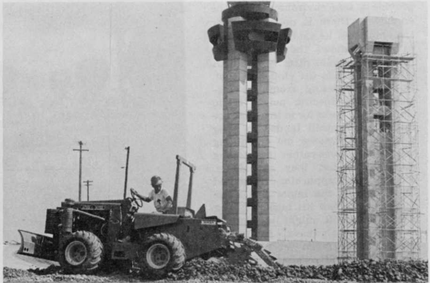
About 65 miles of trenching were accomplished. The Dallas/Fort Worth Airport lays claim to the world's largest non-ag irrigation system.
