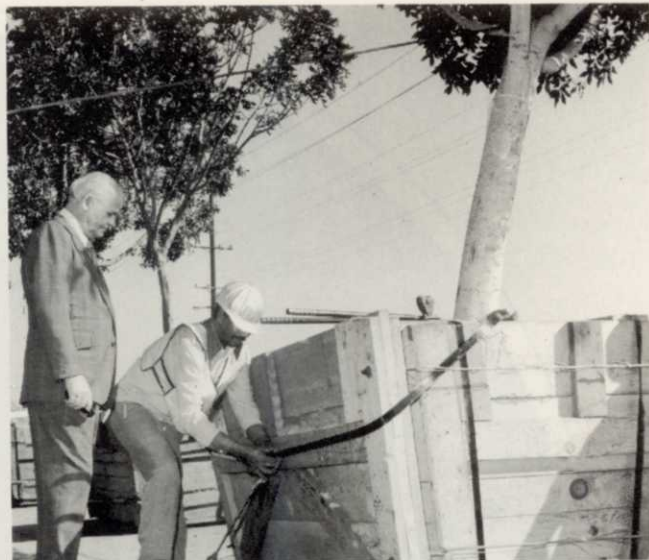
Anahiem Mayor Jack Dutton (l) watches as one of 52 trees is boxed for removal to city parks. Jori Cervantes adds final strapping to an Indian Laurel. Another 55 trees will be saved from two other road widening projects.
