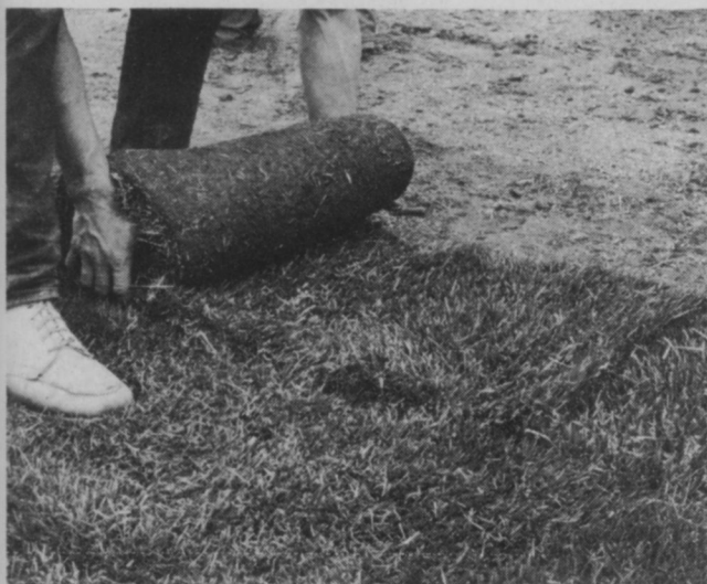
Strips of sod are rolled down end to end to create an "instant" lawn. In a few short hours a bare area can become a site of beauty.
