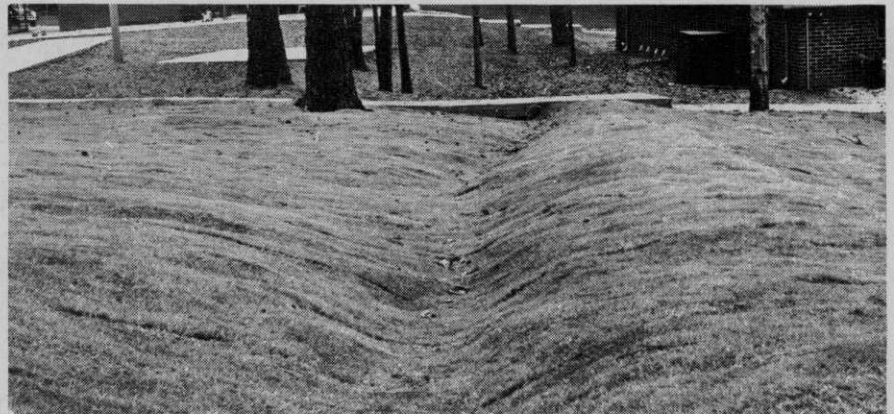
7. Trees, sidewalks and ditches presented no problem on this job which was laid by an inexperienced crew.
