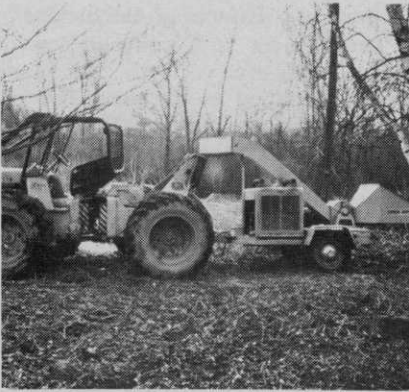
In selective initial clearing, chipper is used to help handle brush.
