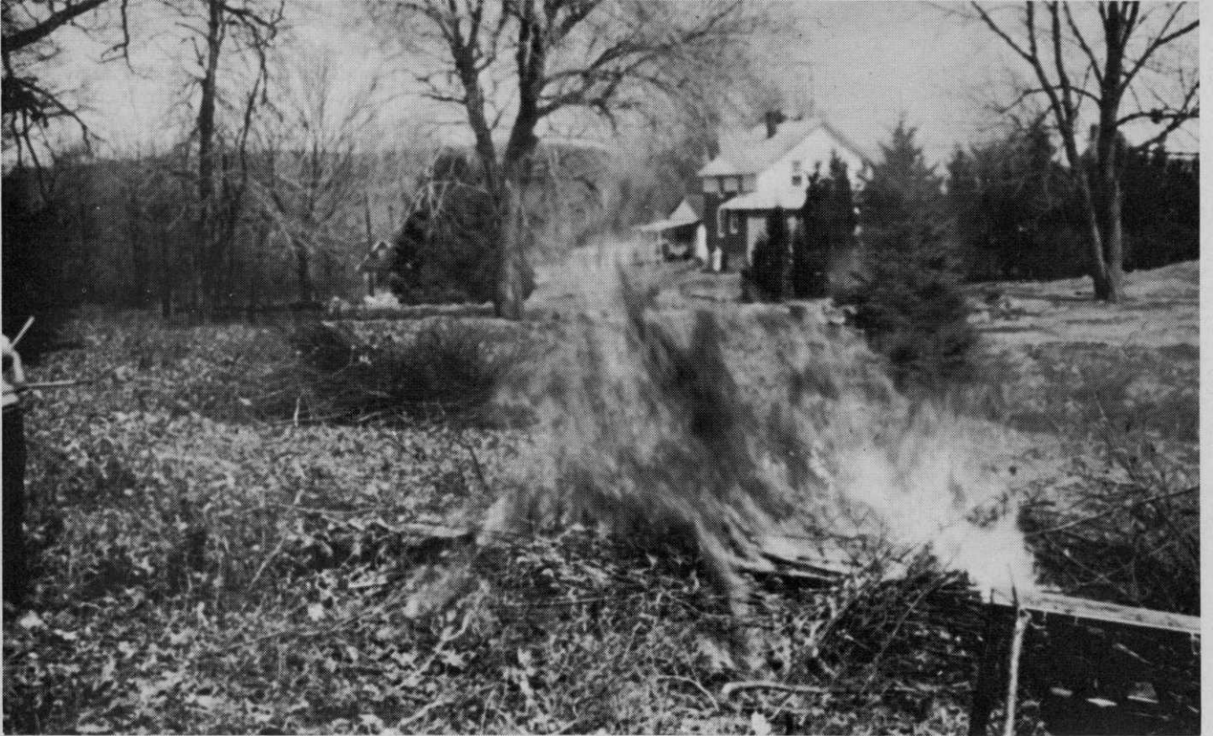
Northeast Utilities burns cleared brush using fanned air and kerosene to intensify burning with less air pollution.
