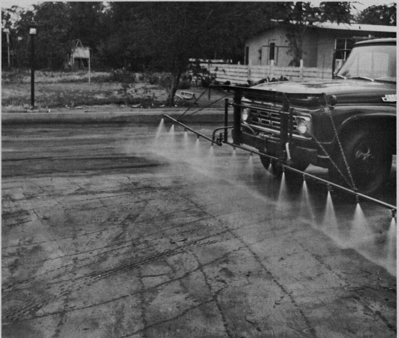
A typical parking lot is bladed to remove existing weed growth and compacted for better surface — prior to application of herbicide and asphalt. Pramitol 25E is applied on the \frac{1}{3} -acre parking lot below in less than an hour, with difficult areas sprayed by hand.
