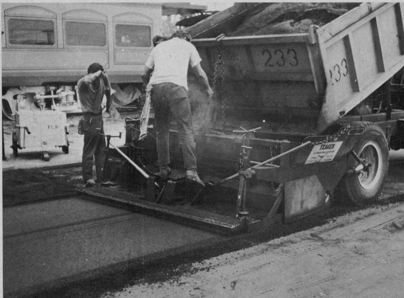
An hour after herbicide was applied to the parking lot, an asphalt crew went to work. The herbicide used is designed to cling to soil particles and not leach out from under asphalt. As a pre-emergence it is used to kill weeds before they are large enough to damage asphalt.
