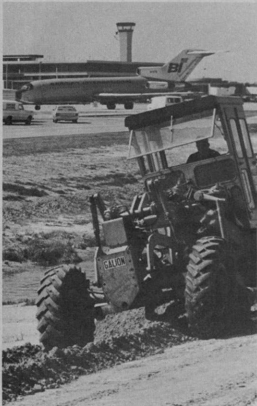
Houston uses a road grader to improve drainage ditches.
