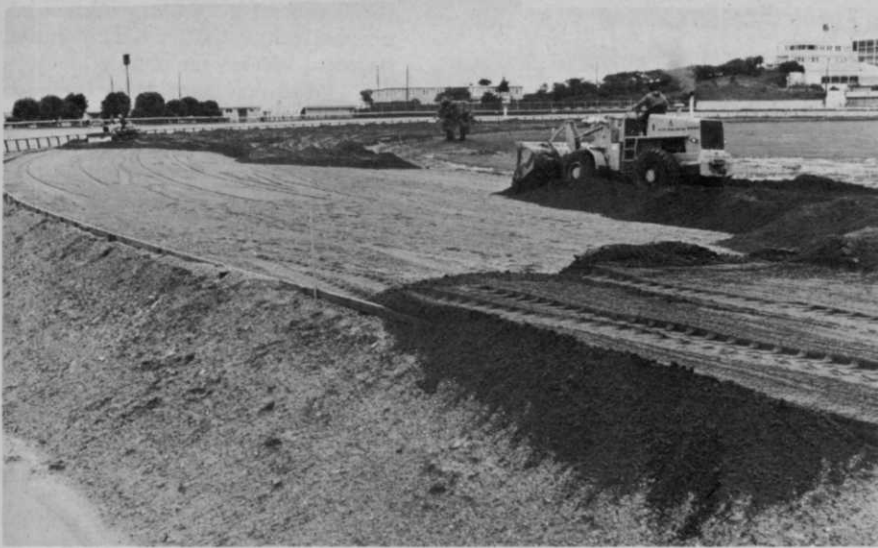
More than 5600 cubic yards of Vita-Bark nursery mix is being used for building the first turfgrass race course in Northern California at Golden Gate Fields, Albany. Planting material being used is one-third Vita-Bark Nursery Mix, two-thirds washed sand, and commercial fertilizer. Grass will be seeded in February. The bark mix is made up of 90% pure bark from white fir, red fir, and pine. Material is passed through a quarter-inch screen and contains nitrogen, iron and a non-ionic biodegradable wetting agent. For more details, circle (717) on the reader service card.
