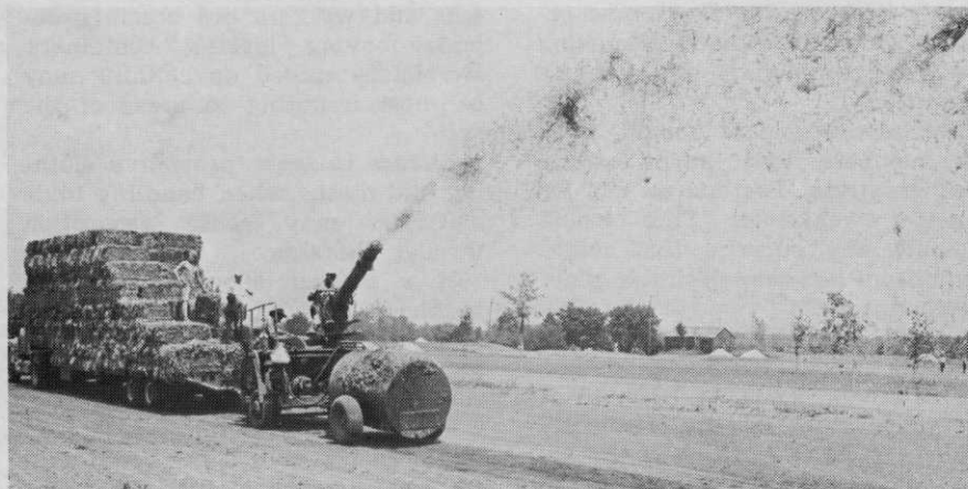
Mulch was spread after seeding to retain soil moisture and assure maximum germination.
