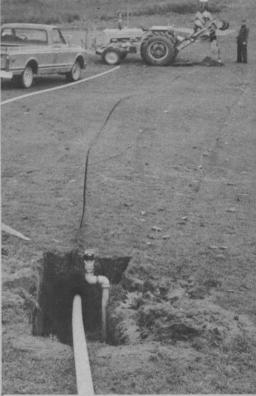
while Flintite Corp. produced the asbestos variety. All the pipe 3 inches in diameter and smaller, the majority of the system, was plowed in with the DP-30 Saber Plow. For the remaining large diameter pipe, Soderstrom used a Parsons 150 trencher and backfilled with a Case dozer. In all, a total of 16,000 feet of pipe was installed.
