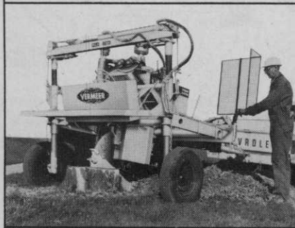
MODEL 1560 — This one has 60 hp Wisconsin engine. More speed and more power for heavier work loads. Cuts 24" deep. Great for land clearing.
