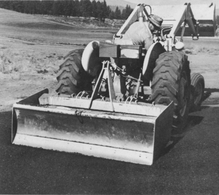
Preliminary rough grading of the Graeagle Meadows golf course greens and tees involved spreading fir bark four inches deep over a 14-inch layer of washed sand. The bark replaces peat.
