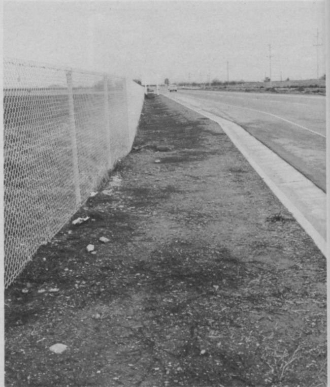
Clean shoulders on modern superhighways are kept weed-free with short-residual herbicides that enable landowners to plan housing or industrial developments without limitation.
