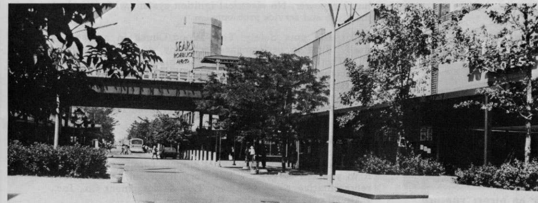
Englewood Shopping Concourse, Chicago, Ill.
