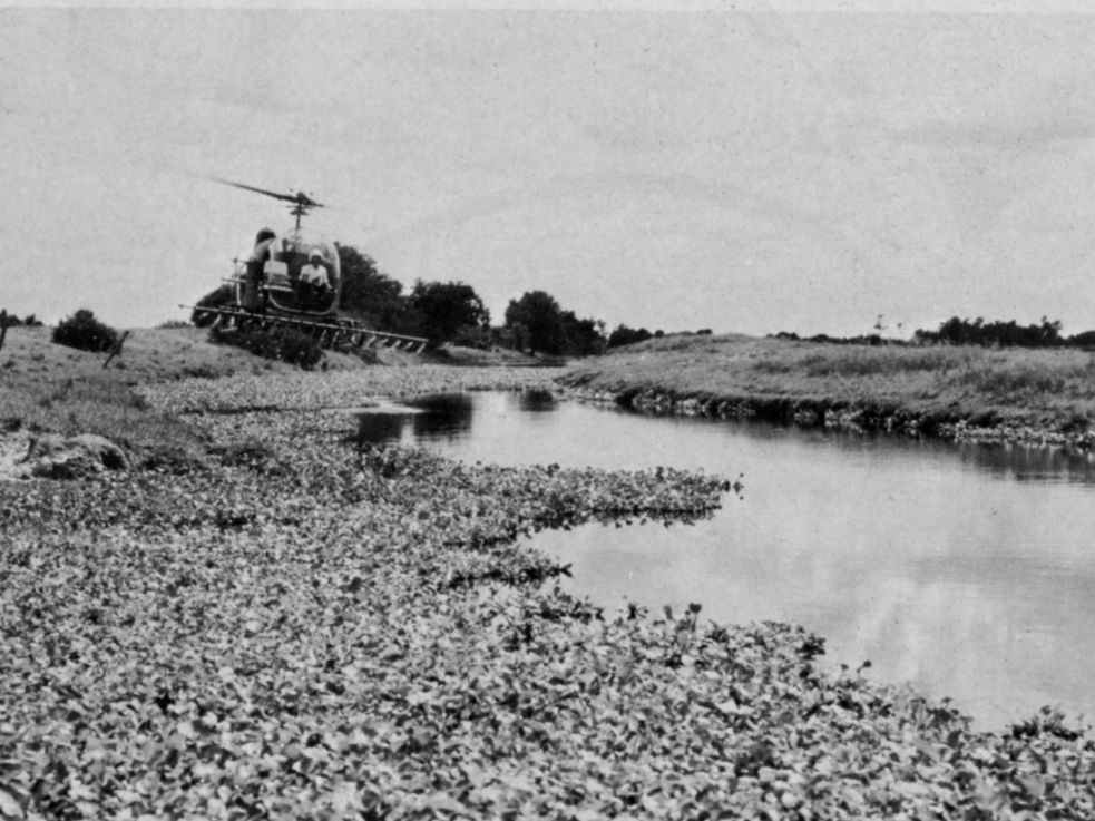
Spraying herbicides on aquatic weeds to keep canals and drainage ditches open, especially in low lying areas, has proved a job made to order for the helicopter. Above, Perdue sprays hyacinths in drainage canal.
