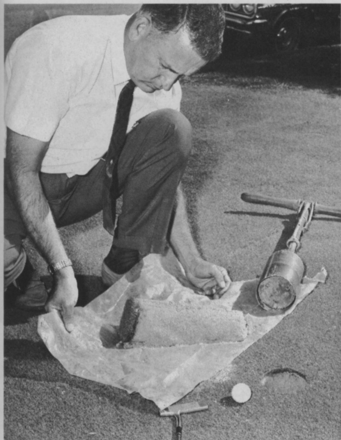
Plastic sheets buried 20 inches below ground level save moisture for golf green turf. Dr. W. H. Daniel, above, Purdue University turf specialist, examines core of turf-topped sand from test golf green. Plastic laid beneath ground surface serves as a "stopper" for moisture. Daniel says this is similar to the old kerosene lamp idea. The plastic barrier serves as the container, and water rather than kerosene seeps up through the sand which is the wick and helps maintain a healthy turf. Coarseness and depth of sand can be varied, according to Daniel. He finds that turf stays moist and green longer, needs less water, and develops deep roots. Also, the turf wears well. He suggests the barrier may be equally practical on athletic fields.
