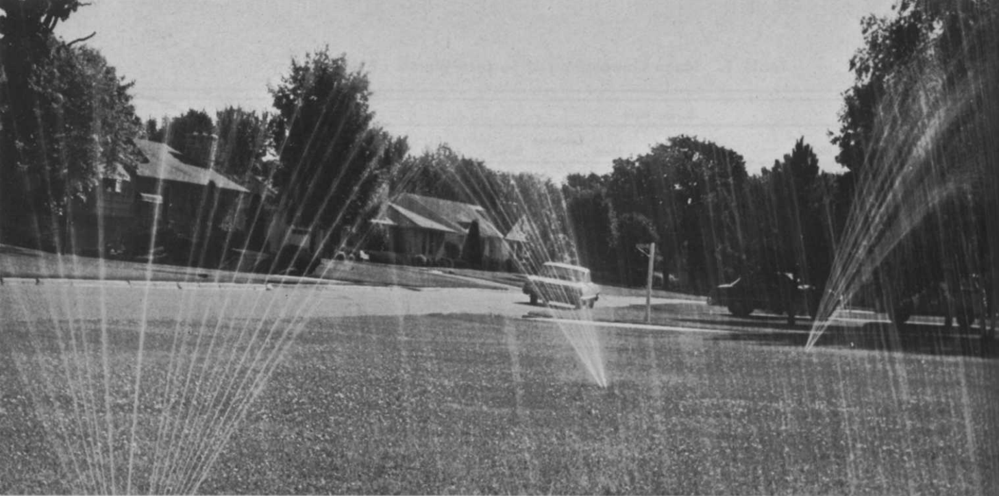
Small neighborhood park is being irrigated with an efficient wave-type sprinkling system. (Its control box is shown below.)
