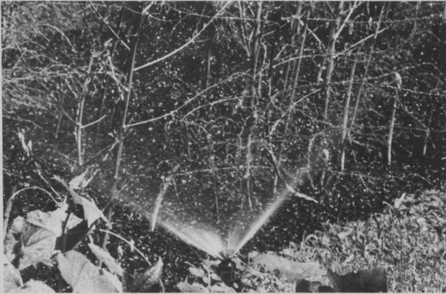
This pop-up sprinkler is directing water away from the leaves.
