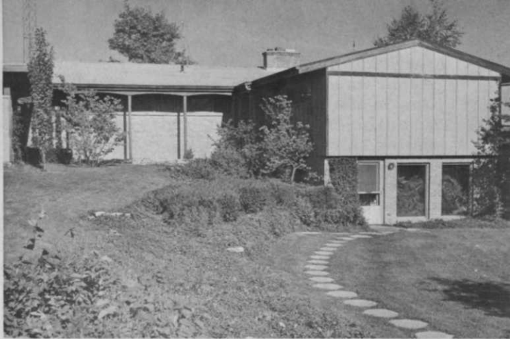
New and modern dwelling is designed specifically for both home and business. Entire ground floor is used as office headquarters for the 7 divisions of the company.
