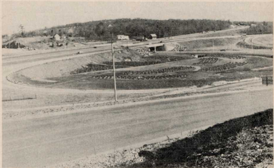
Example of formal planting in the Massachusetts program is this interchange located at intersection of Routes 128 and 37 near Braintree. Joseph L. Beasley, Department of Public Works, reports that bridge abutments, including bed plantings and individual trees are mulched with 3 inches of wood chips.
