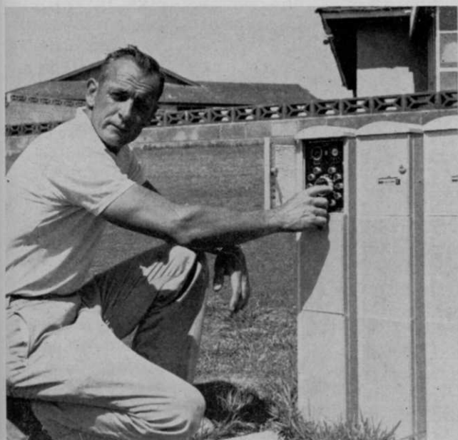
Control box for automatic irrigation system permits control of water applications with a minimum expenditure of time. Conservation of water and higher quality turfgrass are additional benefits cited for automatic irrigation systems.
