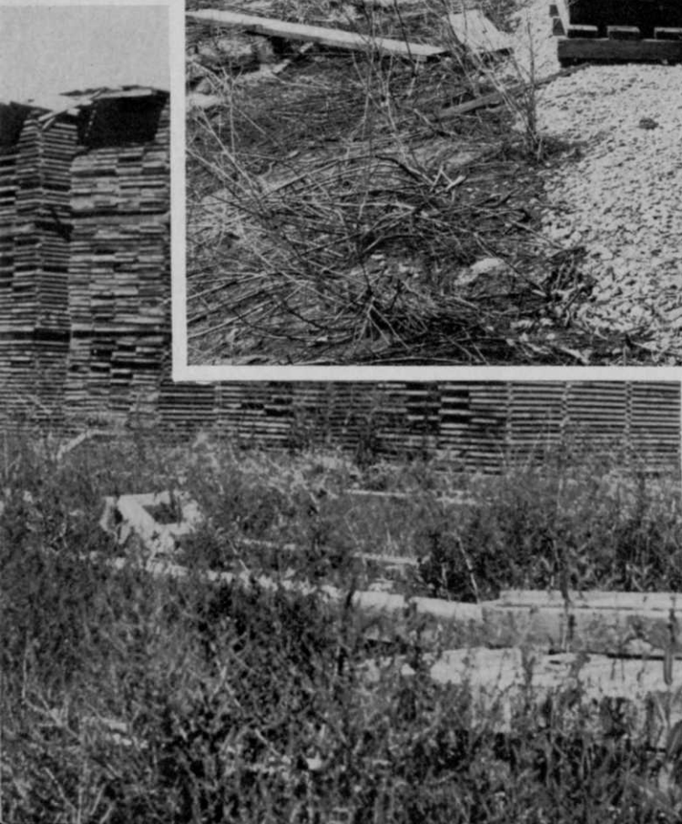
Uncontrolled weed growth in lumber yard (left) is unsightly, creates a potential fire hazard. Above, application of an industrial herbicide at this site killed weeds, still seen beyond chain link fence.
