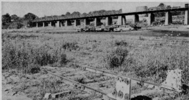
This railroad siding was infested with fire-hazardous vegetation before "Hyvar" X bromacil weed killer was applied. "Hyvar" X controls perennial weeds and grasses (such as Johnson, Bermuda, nut, horsetail, plaintain, wild carrot and bouncing bet).
