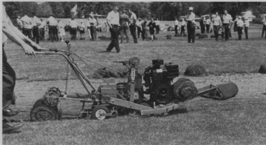
Hadfield Sod Roller , designed to fit on Ryan sod cutter, was among new equipment demonstrated. Hadfield reports unit operates strictly as 1-man operation and is particularly well adapted to smaller sod farm. Roller is manufactured by Hadfield at Oxford, Mich.
