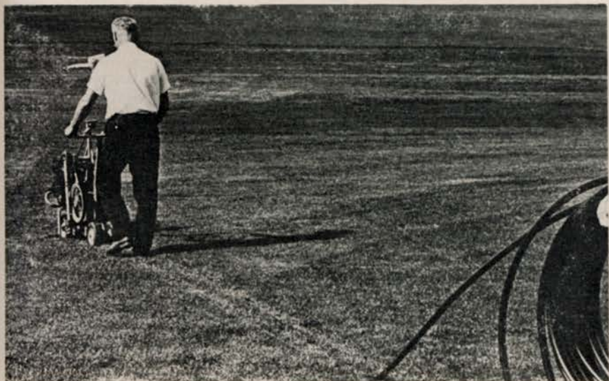
"Mole" leaves only a narrow slit in the turf as proof of its work. The slit quickly disappears, though, and there is no trace that Ryan's "Mole" has installed underground pipes, cables or tubes.
