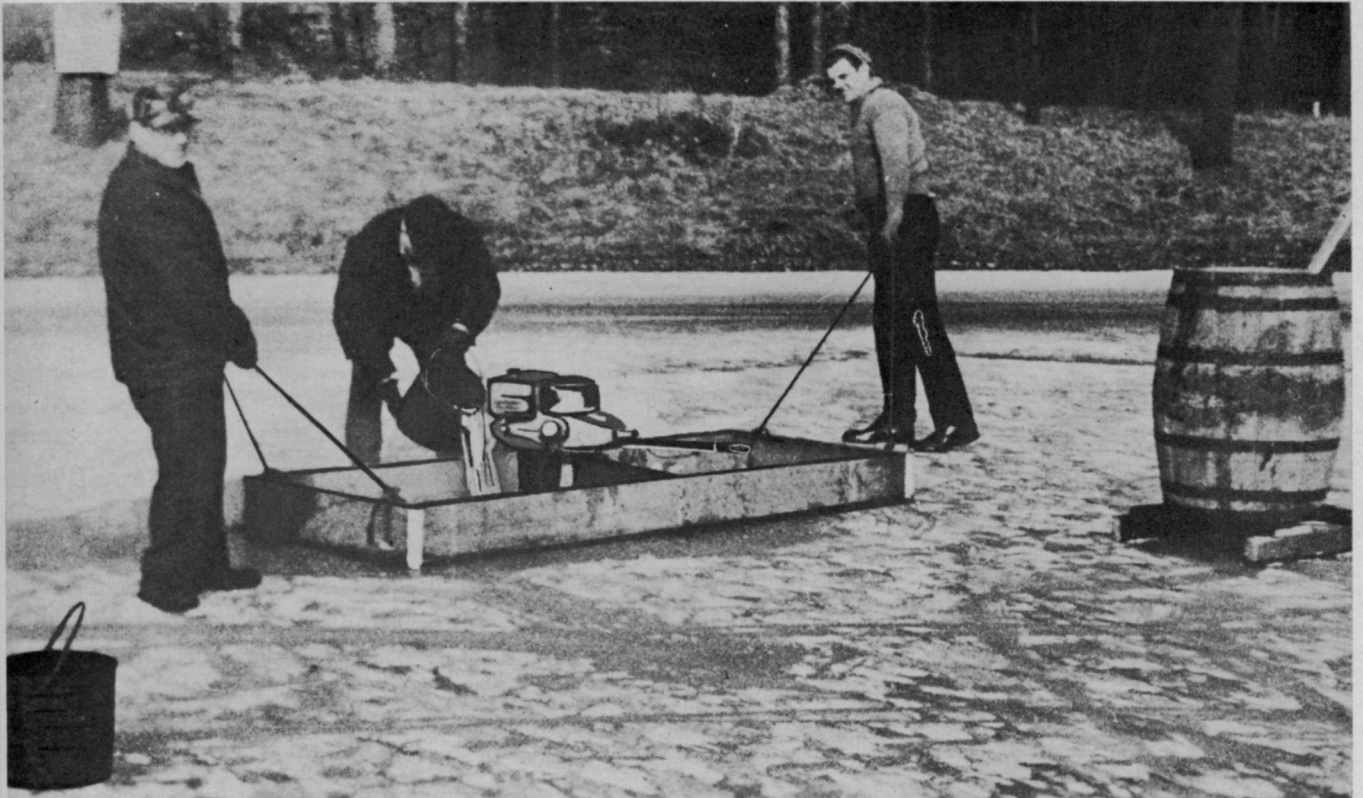
Employees of the Water Division, Massachusetts Metropolitan District Commission, treat for algae under ice. Copper sulfate solution is poured through hole in ice into current generated by outboard propeller. Rotating the complete frame 360°, effectively dispenses the algicide in an area 100' to 150' in diameter. With such a rig a reservoir of 50 to 80 acres can be treated in a minimum of time. Barrel on right holds algicide.
