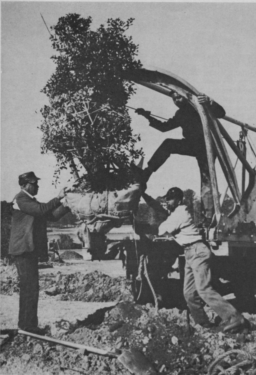
Callaway Garden's "A Frame" tree mover is shown here transplanting large Burford Holly.
