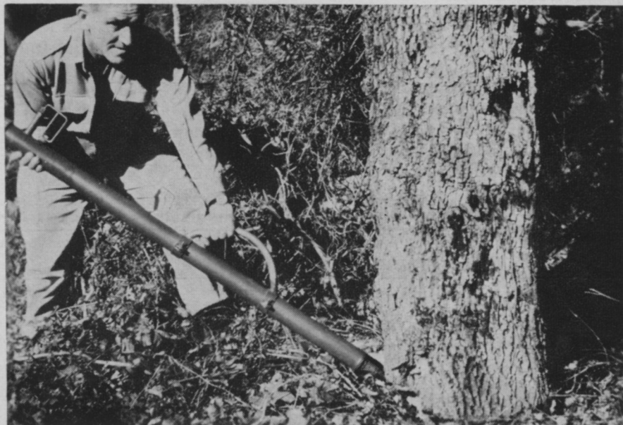
Danger trees are removed from TVA grounds by using a tree injector which is filled with chemicals to remove unwanted, hazardous trees.
