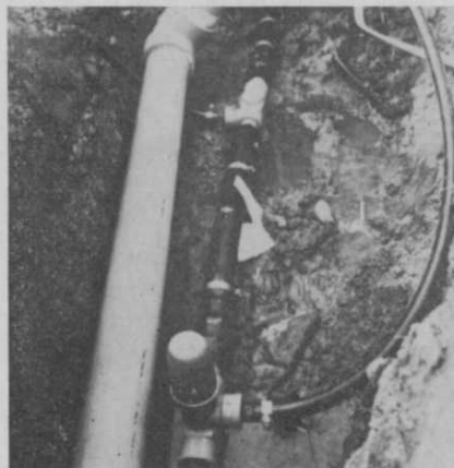
Using the Sequa-Matic valve in a circuit-by-circuit sprinkling system requires the use of only one solenoid valve for the entire system, John Bean says.
