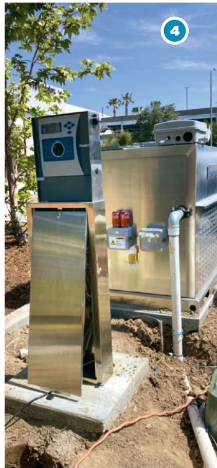
1. A 24-inch-deep trench for the recycled water mainline was at the core of water management at Citrus Commons. 2. Steel supports for a floating walkway that was utilized throughout the property. 3. Catch basins and storm drains direct runoff to the storage tanks to be recycled as irrigation water. 4. An irrigation controller from Hunter manages the entire system.
