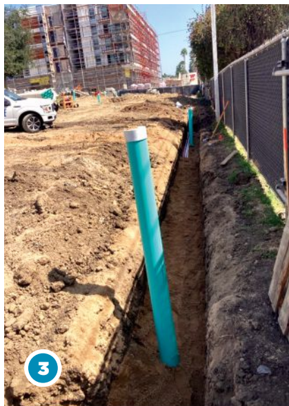
1. A 24-inch-deep trench for the recycled water mainline was at the core of water management at Citrus Commons. 2. Steel supports for a floating walkway that was utilized throughout the property. 3. Catch basins and storm drains direct runoff to the storage tanks to be recycled as irrigation water. 4. An irrigation controller from Hunter manages the entire system.
