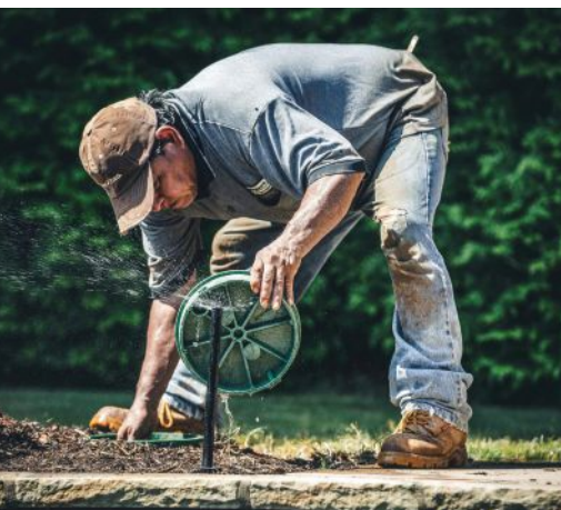
A contractor should make checking items for wear a top priority during regular maintenance.
