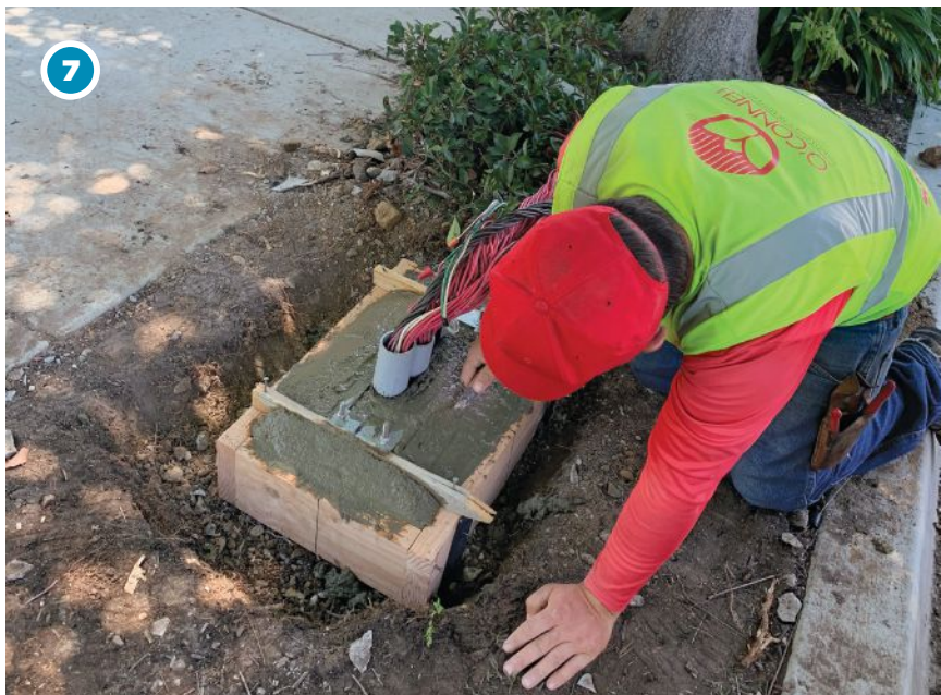
PHOTOS: O'CONNELL LANDSCAPE MAINTENANCE
