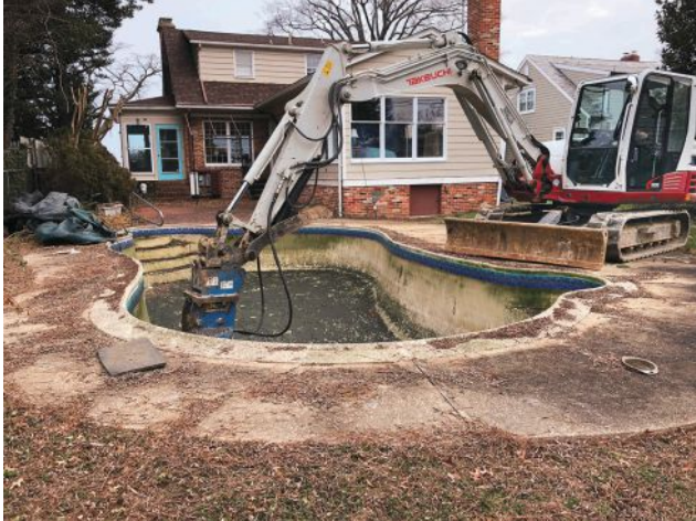
Left: Carroll Bros. Contracting removes a swimming pool from a client's backyard with the Takeuchi TB285 Compact Excavator in the winter. Right: Same backyard later that spring, after demolishing and filling the swimming pool.
