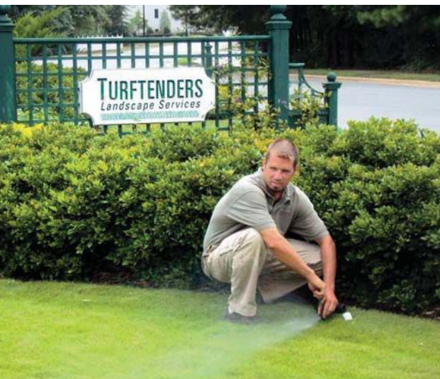
At left: Josh DeMoll, irrigation technician, sets an irrigation head. Below: A Turftenders' account undergoes an irrigation audit.
