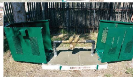
Security cages protect clients' irrigation backflow devices from thieves, who steal the equipment to sell it as scrap metal.
