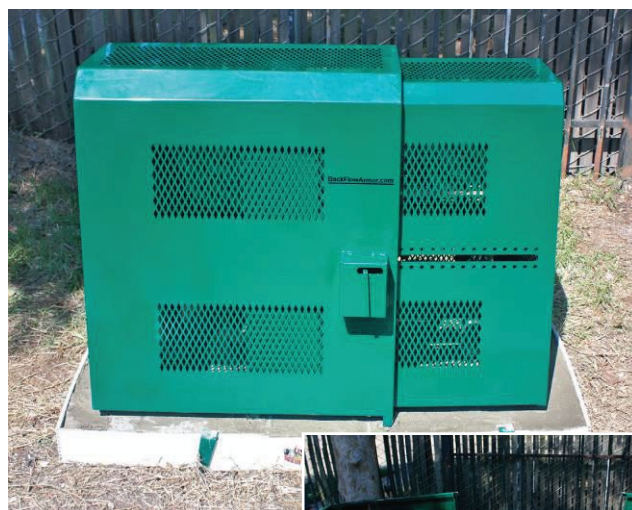
Security cages protect clients' irrigation backflow devices from thieves, who steal the equipment to sell it as scrap metal.
