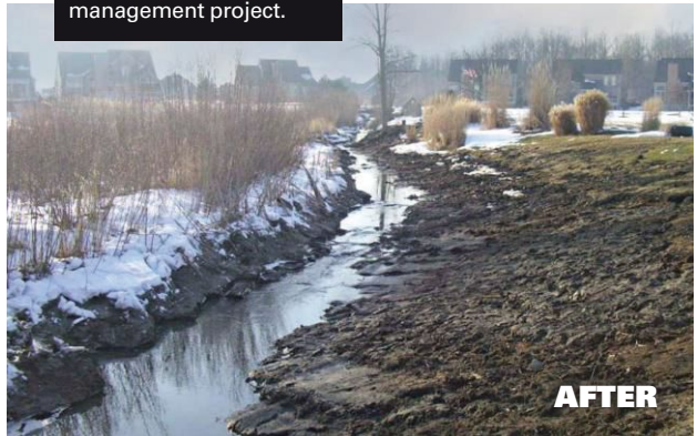
A before-and-after look at a Twin Oaks stormwater management project.
