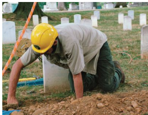
A volunteer installs cables to help protect trees from lightning strikes.
