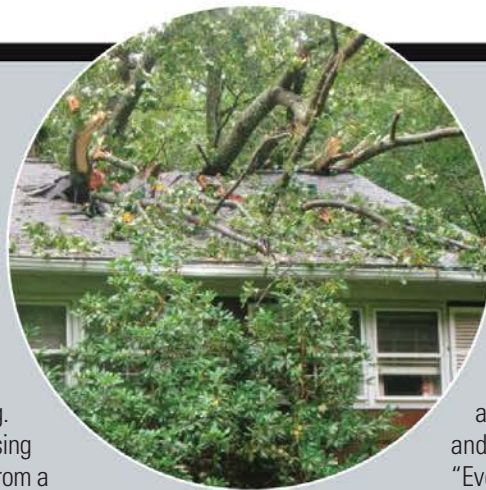
A tree smashed through the roof of a home in Trumbull, CT, near Stamford.
