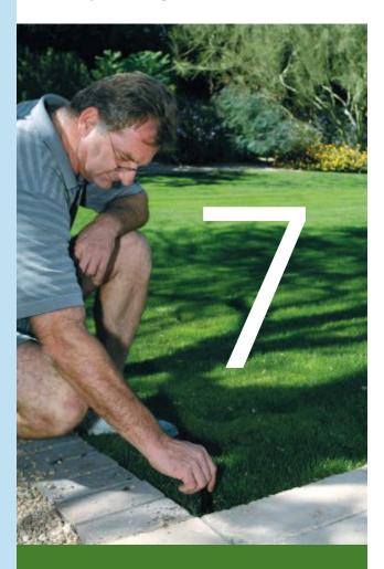
Adjust arcs. Just as you properly flush the system so you do not get clogged nozzles, take the necessary time to adjust the sprinkler arcs so they're properly watering what they're intended to water. Make sure none of the arcs are watering the hardscapes. Every time you have to come back to adjust something, it costs you money, but it also shows the general contractor and/or the owner that you didn't install the job properly.
